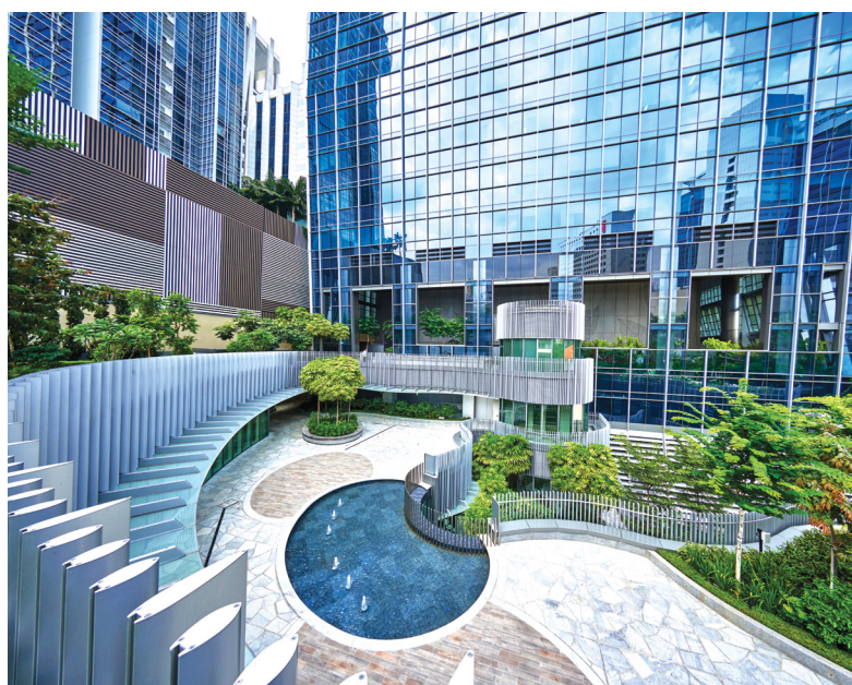
▲ Frasers Tower • Singapore
