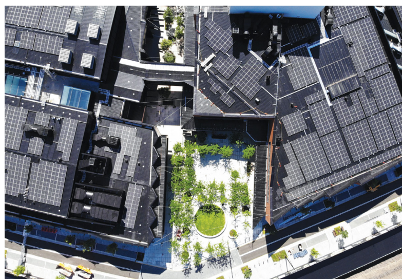
▲ Solar panels at Ed.Square Town Centre, New South Wales • Australia
